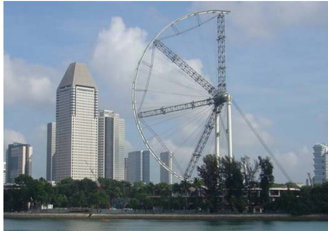
Figure 7 : View looking North West during erection
